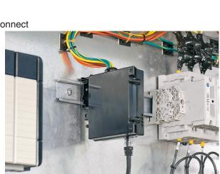
Isolation module can be mounted to DIN rail (shown) or mounted to surface using provided mounting tabs.
